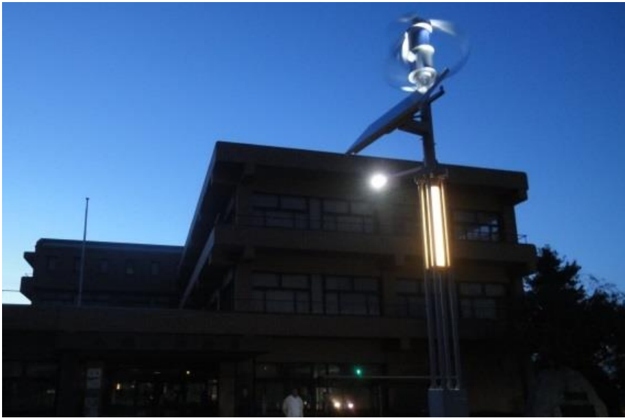
Wind solar hybrid system for parking lot lighting, Ibaraki, Japan
