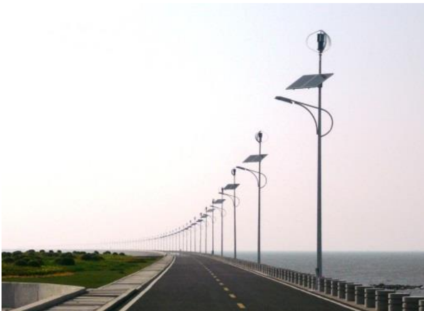
Wind solar hybrid system for road lighting, Shanghai, China
