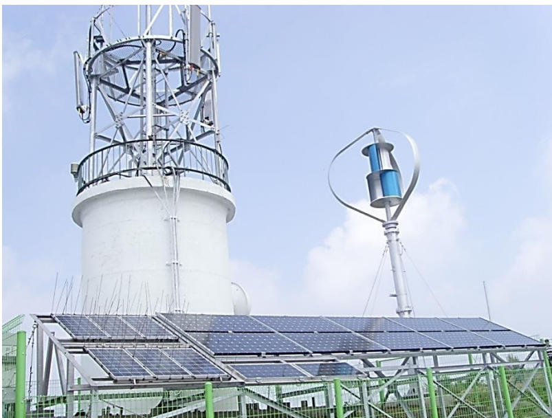
Telecommunication station, Korea
